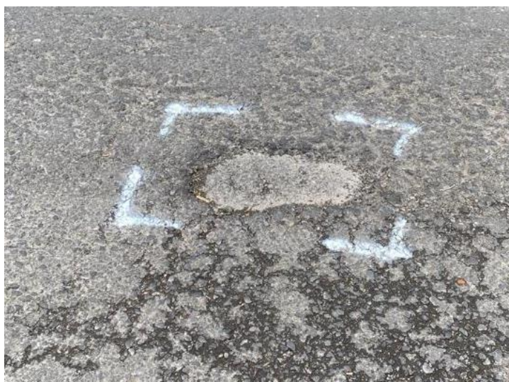
Gambar 1. 2 Lubang ( pothole )
